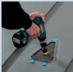
Loch  $\varnothing$  35mm mittig bohren
